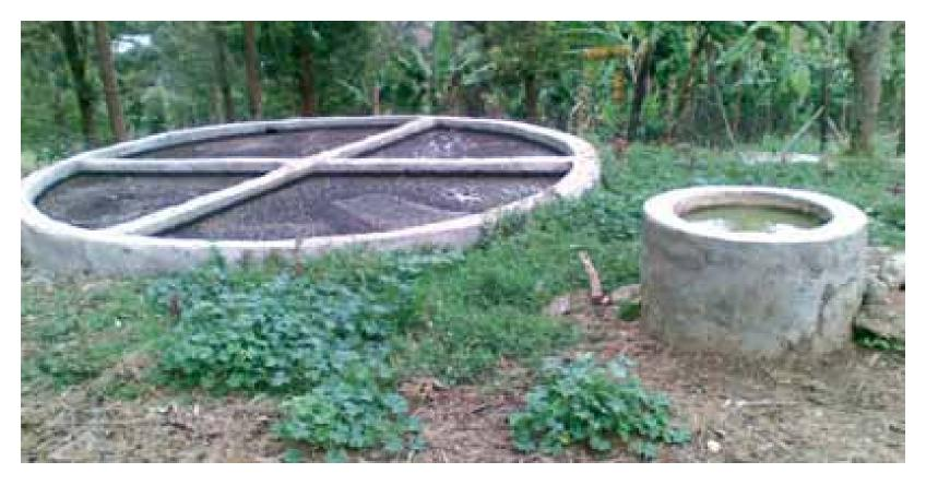
An anaerobic digester and discharge system for biogas generation. Controlled methane
