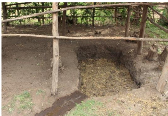
Building a compost pit to improve the handling of bio-slurry.
