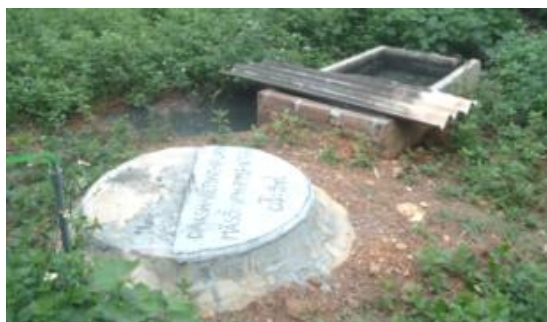
Leaking bio-slurry storage (at top left).
